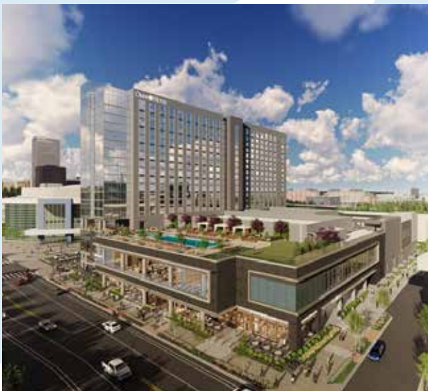
Render picture of Omni Hotel under construction in Oklahoma City
